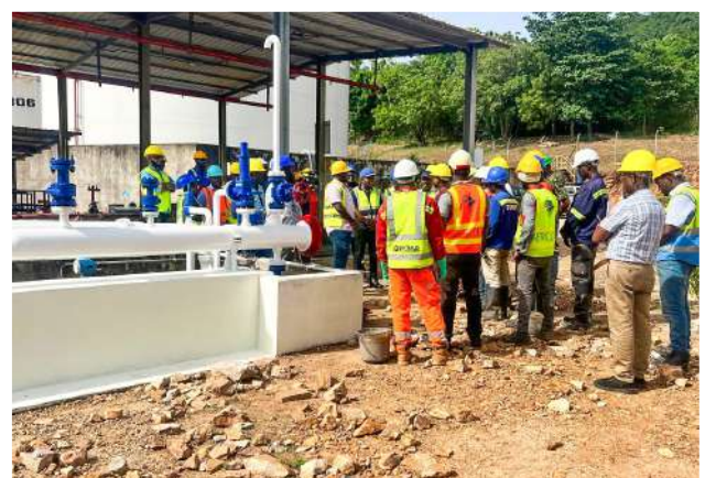
WORKERS RECEIVING THE PIG FROM THE RECOMMISSION TAPP
